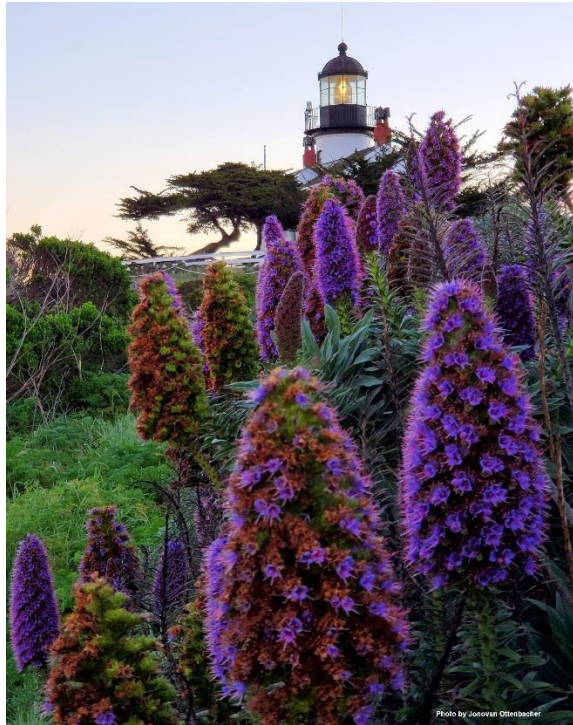
The current Point Pinos Lighthouse light source is a 1 kilowatt bulb, producing a 50,000 candela beam visible up to 15 nautical miles.
